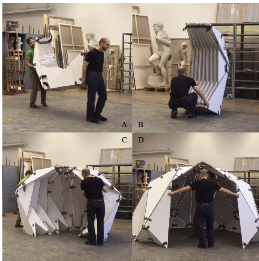
Figure 2: Lightweight, flat-foldable, and cost-effective - origamic structures boast a variety of advantageous properties for exhibition and interior design. Photo: Jiří Palacký.
